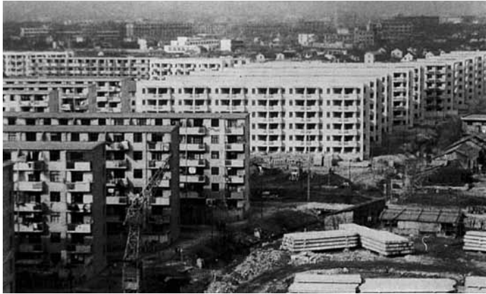
Schiere di case in linea, Cina. Source: Lu Junhua, Zhan Jie, Peter Rowe, Modern Urban Housing in China Ed Prestel 2001 Verlag, Munich, New York, London
